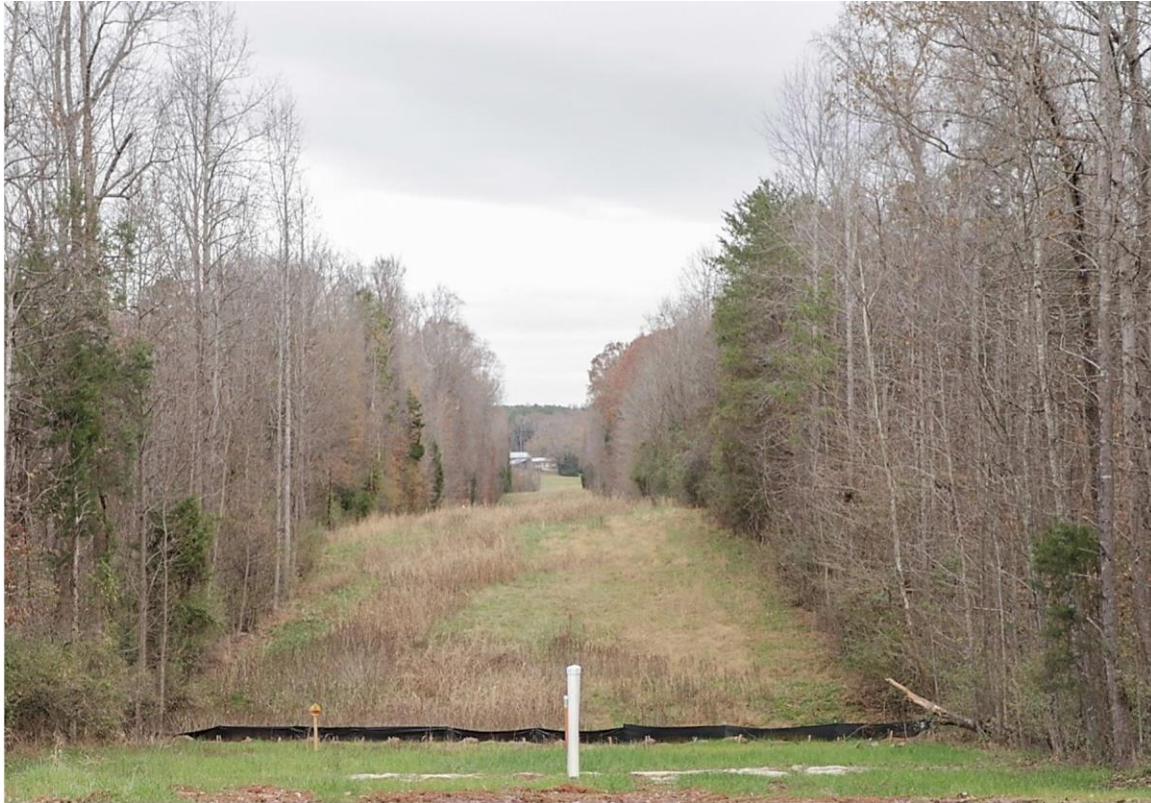
Figure 12. Right of way and monitoring well Colonial pipelines. The lines leaked in Oehler Nature Reserve, Huntersville, N.C. The spill is currently estimated as totaling 2 million gallons of gasoline.
